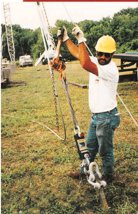
▲ Dyna-Link in use to monitor tower line tension.
