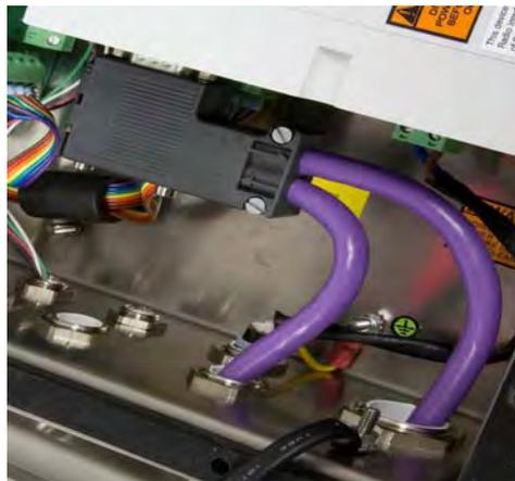
Figure A-58: J-Box Enclosure PROFIBUS Cable Routing
