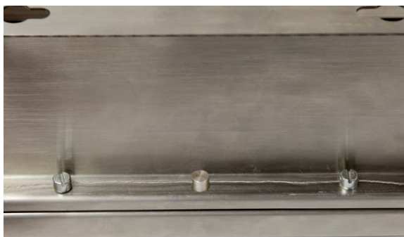
Figure 2-78: Apposition des sceaux version Junction Box (originale) – Goujon et vis de scellage
