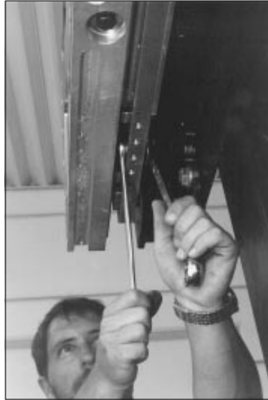
Figure 3b: Adjusting the jam nuts.
