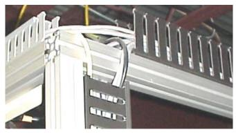
Figure 45: Wiring Channels
